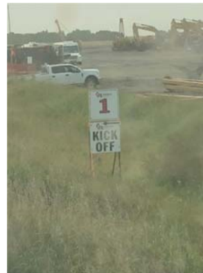
Aug 18/18 congested area at kick off facing East
