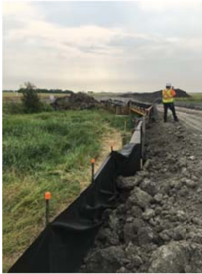
Aug 13/18 Water Course Bridge KP 1000+98 WC #MB-WC58 North side of bridge
