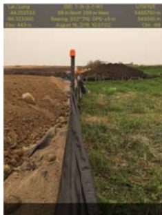
Aug 17/18 Work still in progress, protecting the wetland habitat with geotex and T-posts also the orange mushroom caps being used for safety, facing towards the south
