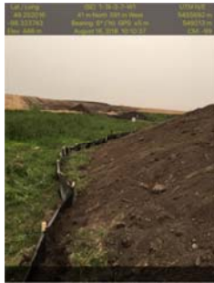
Aug 17/18 Sloped loose soil 12 metres above grade With heavy rain could slide and overcome protective barrier (black with wooden stakes) looking towards north
