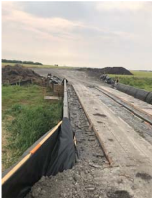
Aug 13/18 Mary Jane Creek temporary man made crossing SSKP 1000.98
