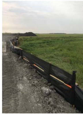
Aug 13/18 Water Course Bridge KP 1000+98 WC #MB-WC58 South side of bridge
