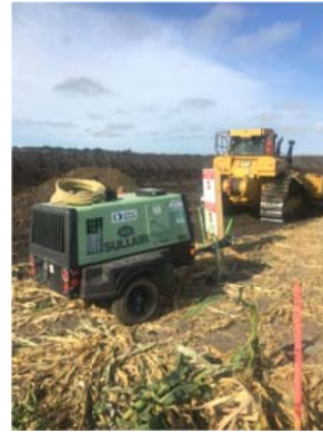
Aug 14/18 Dozer in background grading area for station, compressor will be moved to south boundary opposite from proposed ditch
