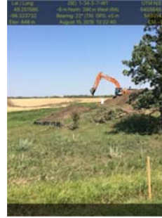
Aug 15/18 Rd#13 KP 1018+800 Work beginning, wetland habitat
