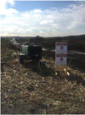
Aug 14/18 Compressor used for cleaning station Rd #9
