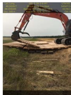
Aug 18/18 Gordie Cardinals Clearing Crew Installing road mats in ditch SA Energy
